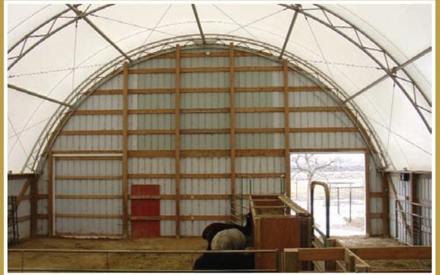
The end-wall of this hoop building has been totally framed up and skinned with metal. The framing allows for easy installation of various door configurations. Note the heavy duty tubular trusses, cable cross bracing and tubular purlins (pipes running between the trusses).
