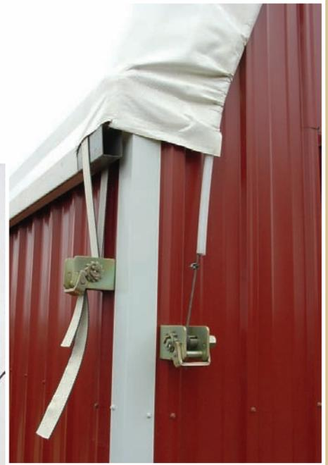
**Above:** The fabric is stretched tight over the top and down the sides of the buildings and also kept under tension by a system of cables, straps and heavy-duty ratchets. The cover is a rip-stop, twelve and a half ounce, twenty-four mil, polyethylene, fabric.
