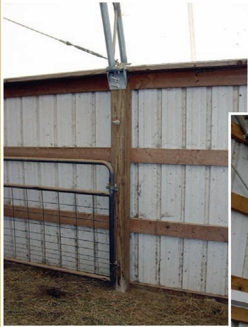
**Above:** The arched trusses of the Post building are bolted to the top of 6' x 6' treated wooden posts, which are set in concrete about four feet in the ground.
