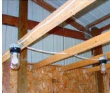
Ceiling joists work great for supporting the ceiling, hanging lights, running wiring, and attaching overhead heaters. The jar lights shown should be used to prevent hot broken bulbs from falling into bedding and starting a fire.
