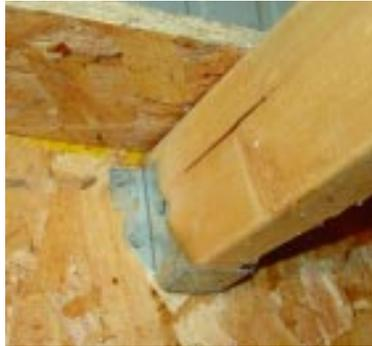
Ceiling joist hangers are perfect for attaching the ceiling.
