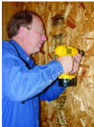
Next, attach the wall covering material such as OSB, plywood, or sheet rock.
