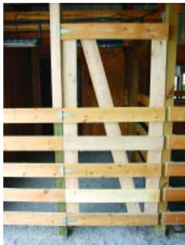
To begin the process of installing a climate controlled stall, first install the posts for doors and the wall supports. Next, attach the board fencing and all doors.
