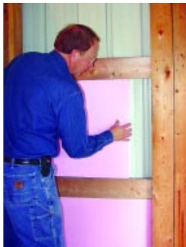
To insulate the exterior walls, you can install solid foam insulation. The top and bottom foam panels are in place. The center foam panel will be added next.
