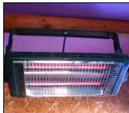
Electric radiant heaters mounted to a low ceiling are safe and efficient for warming crias in wet, cool weather.
