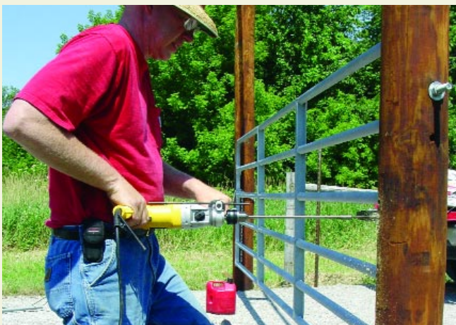
5. Drill holes in the gate post for mounting the gate opener control box. Use caution in locating the control box so that it does not affect the full operation of the gate.
