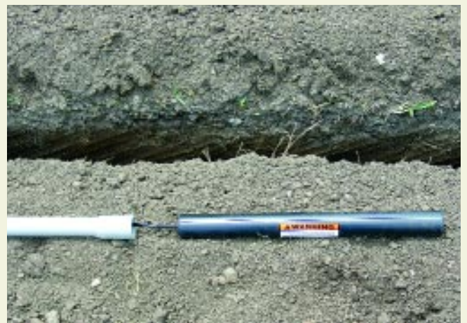
6. A sensor device is available for opening the gate while exiting the ranch. The sensor is installed along the driveway on the property side of the gate, buried about one foot deep and a distance of fifty feet from the gate. When a large metal mass, such as a car, passes near the sensor, the gate opener opens the gate.
