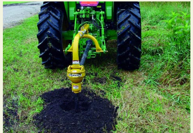
4. Drill post holes and hang the entrance gate.
