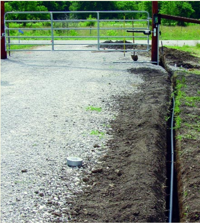
7. Install the exit sensor in the trench and connect the conduit and wire to gate opener control box.
