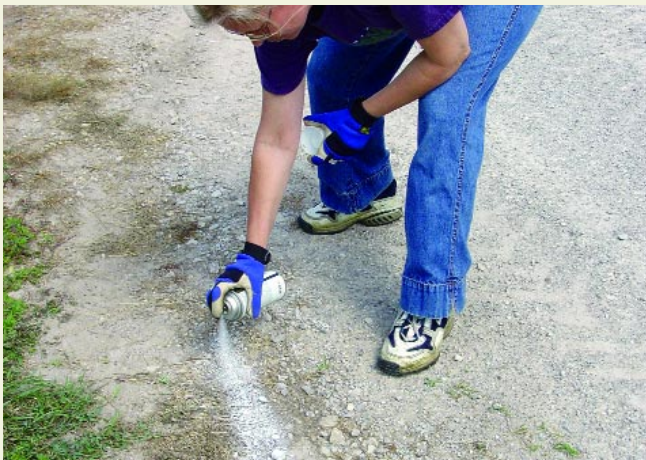
3. Lay out the proposed location for all posts, trenches, etc. by spray painting markings on the ground with white paint. Call the utility companies that serve your area and request they check your spray paint markings and mark their underground utilities prior to you digging.
